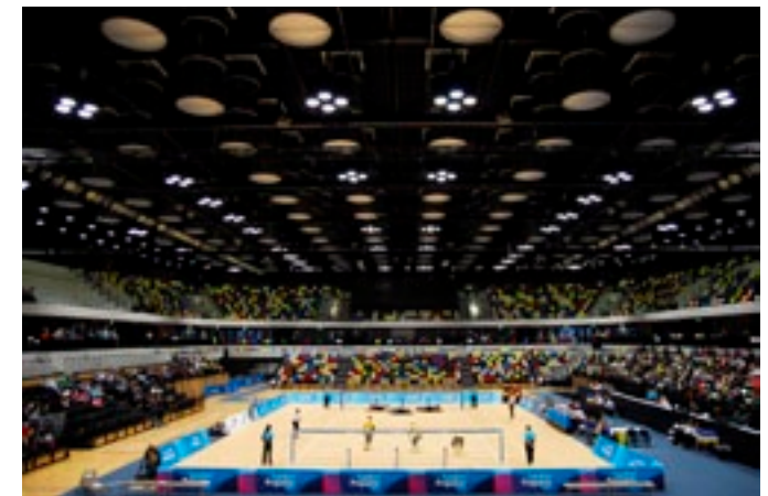
The field of play at the Copper Box is naturally lit through 88 rooftop light pipes
