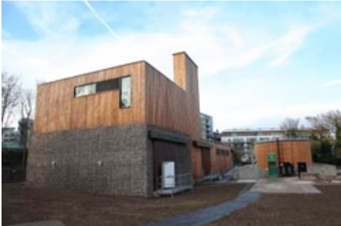
The Old Ford Water Recycling Plant on the Olympic Park provides the largest non-potable water supply network in the UK
