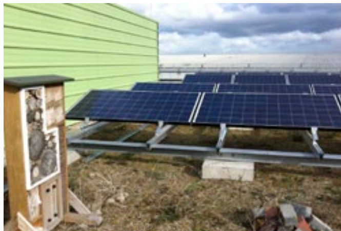
Photovoltaic panels combined with a living roof on the Olympic Park
