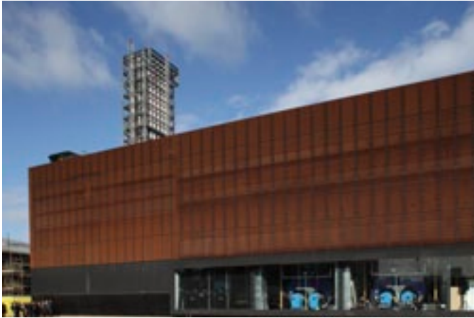
During the Games the Olympic Park Energy Centre will provide efficient, local cooling and heating
